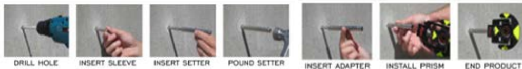
Figure 5. New station installation process
