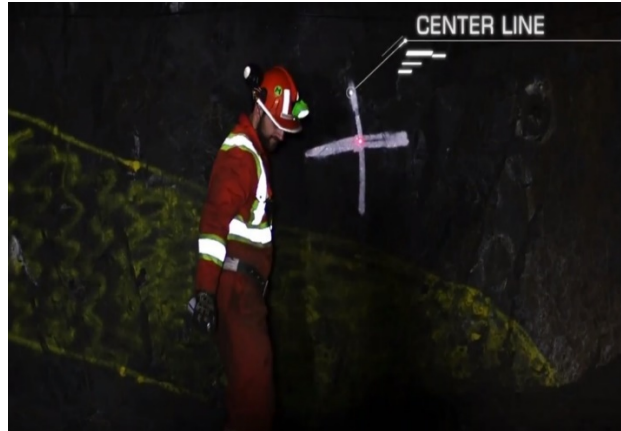
Figure 7. Centerline marked on face
