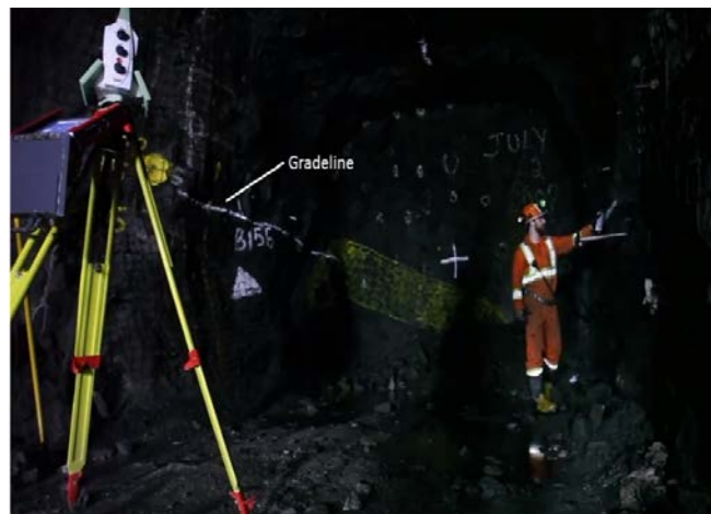
Figure 9. Gradeline being marked up
